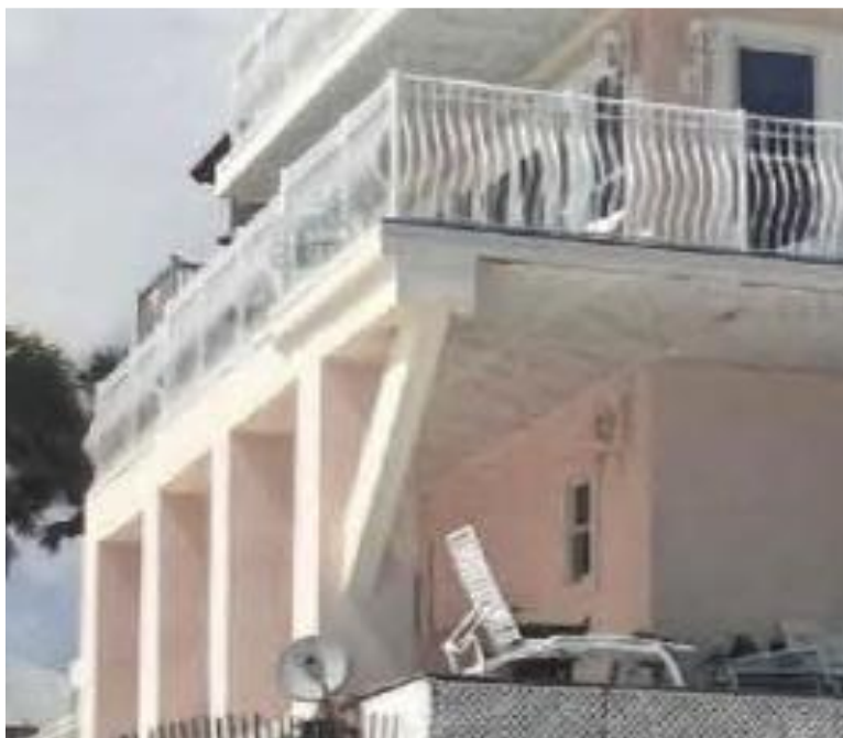
Western deck – before closing and renovations (Doc. 41-3 at 327)
